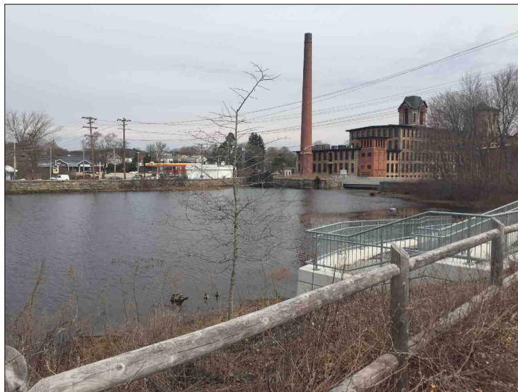
Figure 2: A textile factory along the South Branch of the Pawtuxet River in Coventry, RI.
