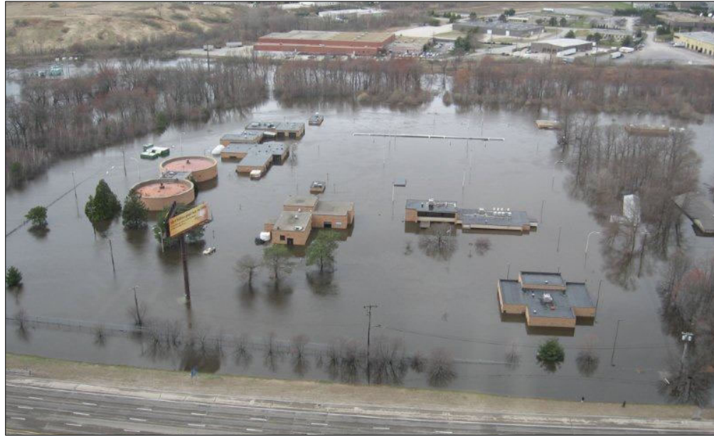
Figure 38: Warwick Waste Water Treatment flooded during spring 2010.
