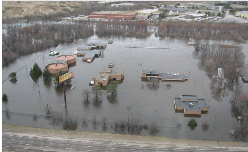
Figure 95: Warwick Wastewater Treatment Facility during the flood in March 2010.
