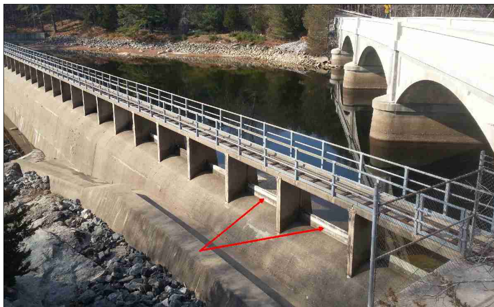
Figure 54: Photo of flashboards in the Scituate Reservoir spillway. Red arrows show the flashboards.
